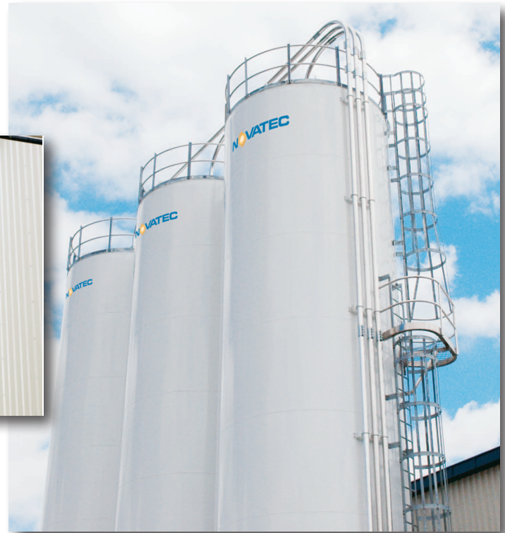
Caged ladders, railings and catwalks
