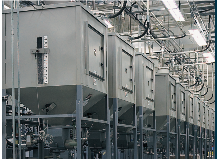
Surge Bin Installation
