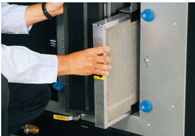
Easily accessed plasticizer filter for cleaning.
