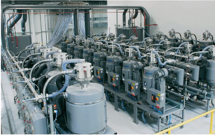
Control of up to 4 central dryers, 48 drying hoppers and 160 material receivers on drying hoppers, blenders and process machines.
