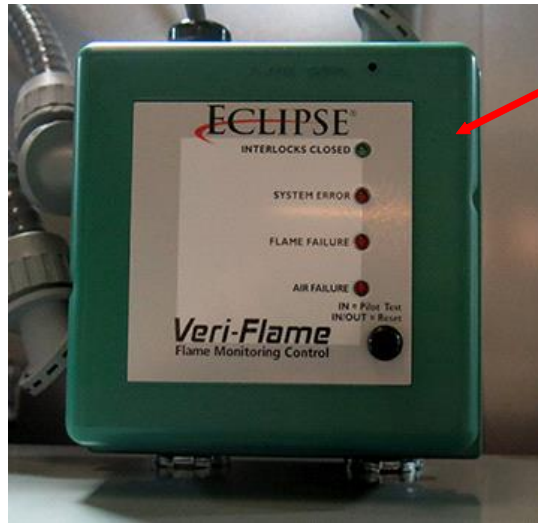
Burner Controller with manual reset and indicator LED's
