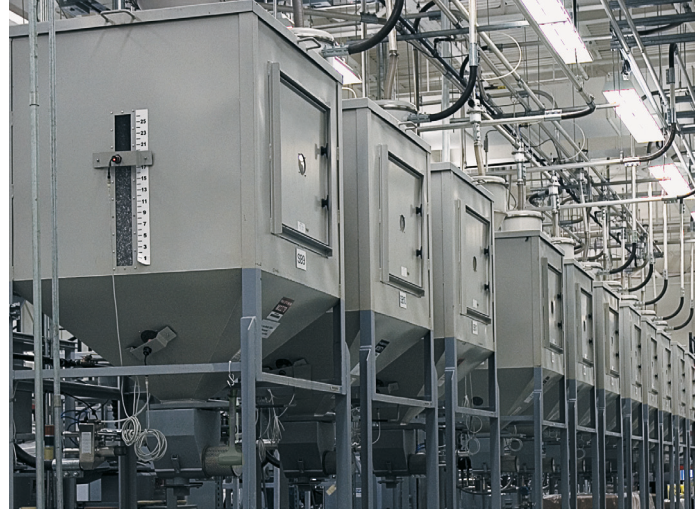
Surge Bin Installation
