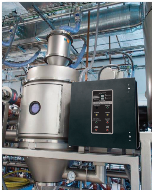
Control locally at CDA2 or from dryer control
