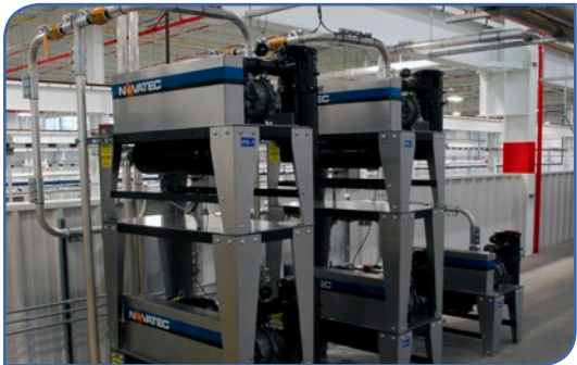
Positive Displacement Pumps Can be Stacked to Save Space
