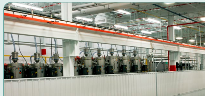
Dryers, Hoppers, Pumps and Material Selection Manifolds on Mezzanine
