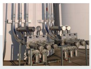
ID proofing gate valves for truck unloading.
