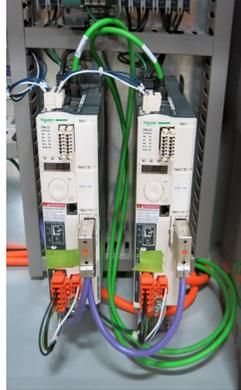
Traction Motor Servo Drives
