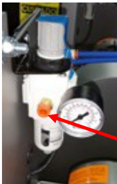
Compressed Air Connection
