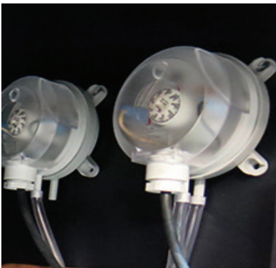
Differential pressure switches can warn of filter clogging.
